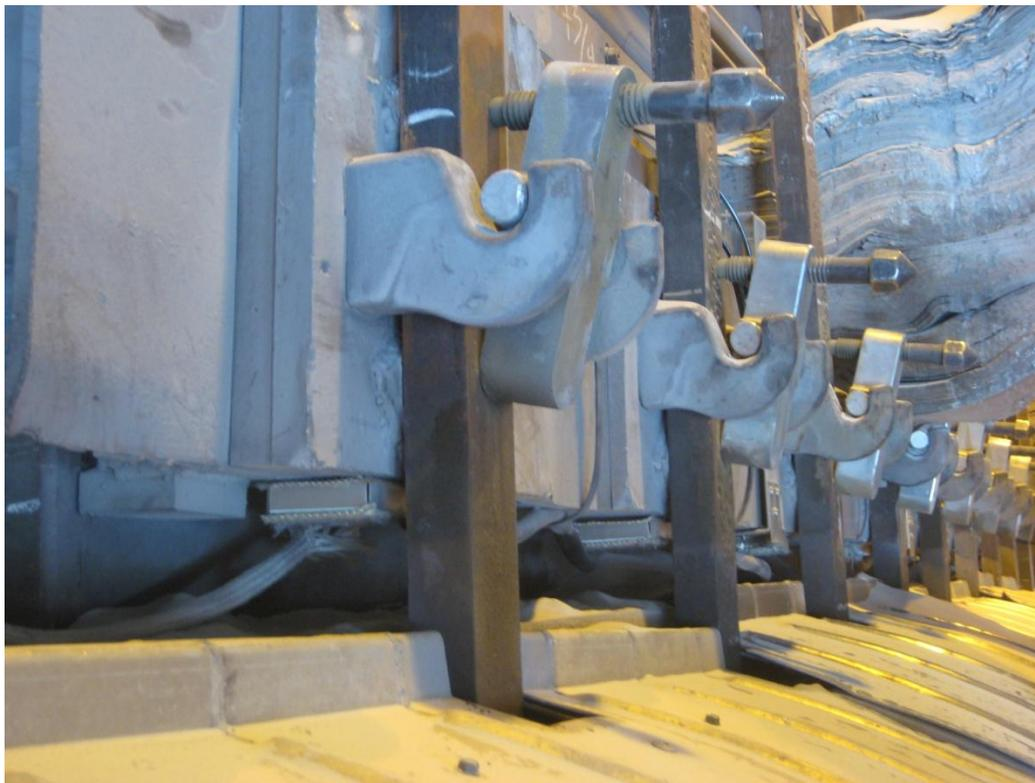
Figure 4. Slaves below the anode beam near the completion of installation.
